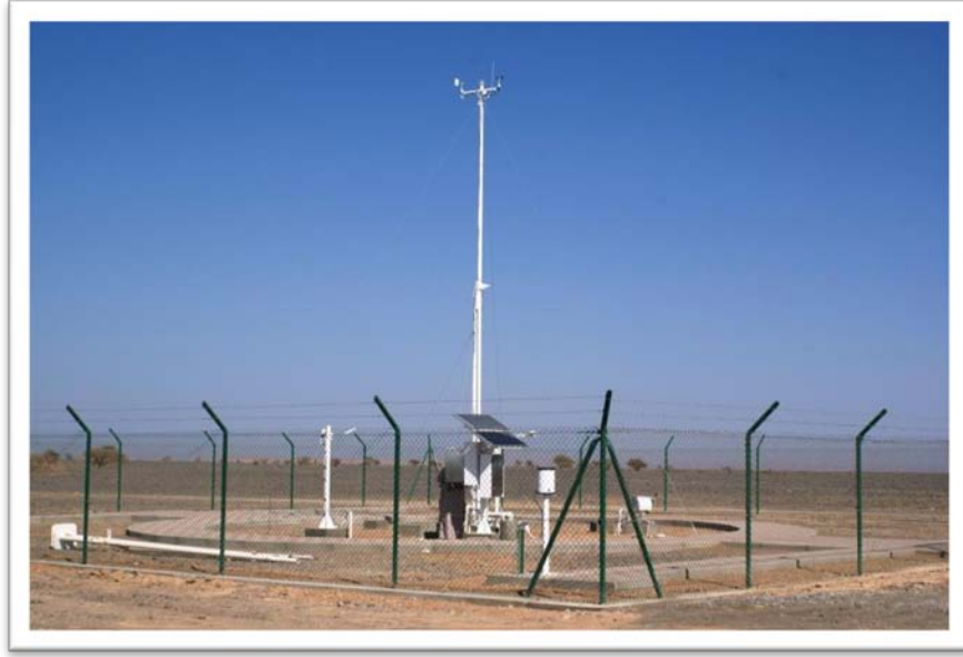
Figure 3-3 Manah Met Station
