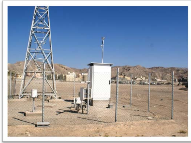
Figure 3-5 Dust Sampler installed at Adam
